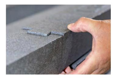
Transfer the length dimension to the assembled profiles.
