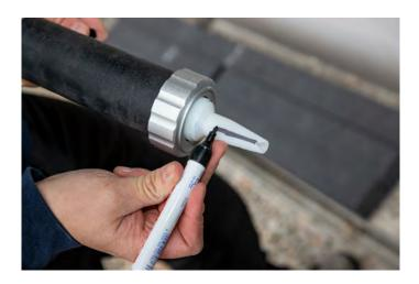
3. Apply the blaugelb Hybrid Polymers Power Fix on the side facing the wall. The two beads must be applied at a sufficient distance from the edge. We recommend applying the adhesive promptly onto all profiles for an opening in the structure.
